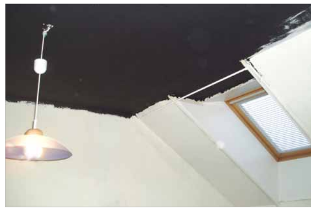
2) Application of HF shielding paint.
